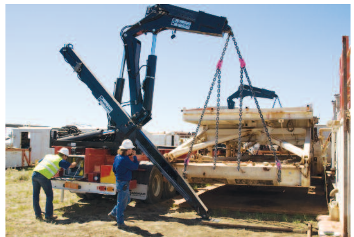
Hammar Rig Lifter loading a 36 tonne sub base
