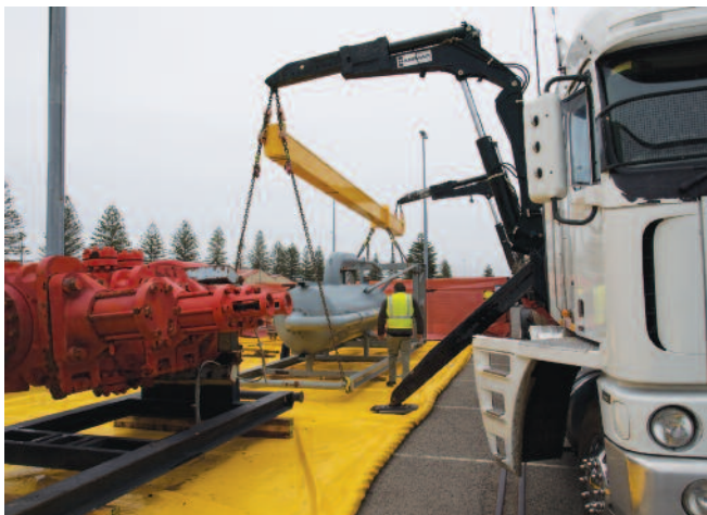
Lifting a degasser directly from the quarantine area
