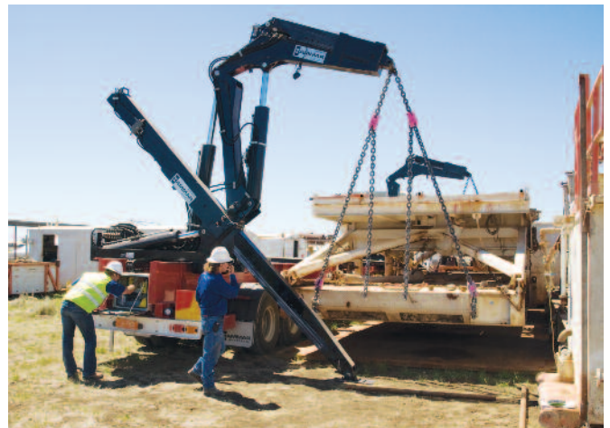
Hammar Rig Lifter loading a 36 tonne sub base
