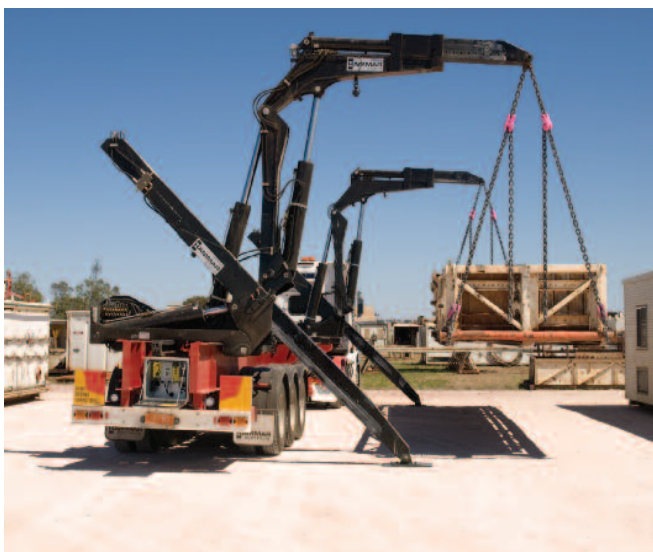
Full pipe bin weighing 20 t being lifted, note reach beyond stabilisers
