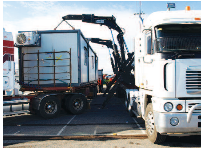
Handling of over length portable buildings
